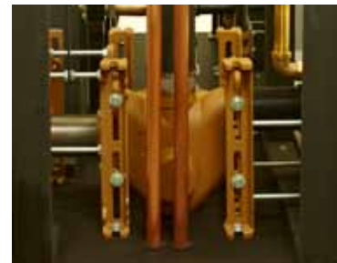
Wall chase images featuring a Fig. # 0240DY-M54 closet support installation.
