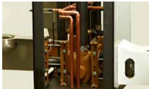
Wall chase images featuring a Fig. # 0240DY-M54 closet support installation.
