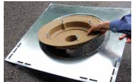
2. Place 1010 roof drain into the sump receiver deck plate.
